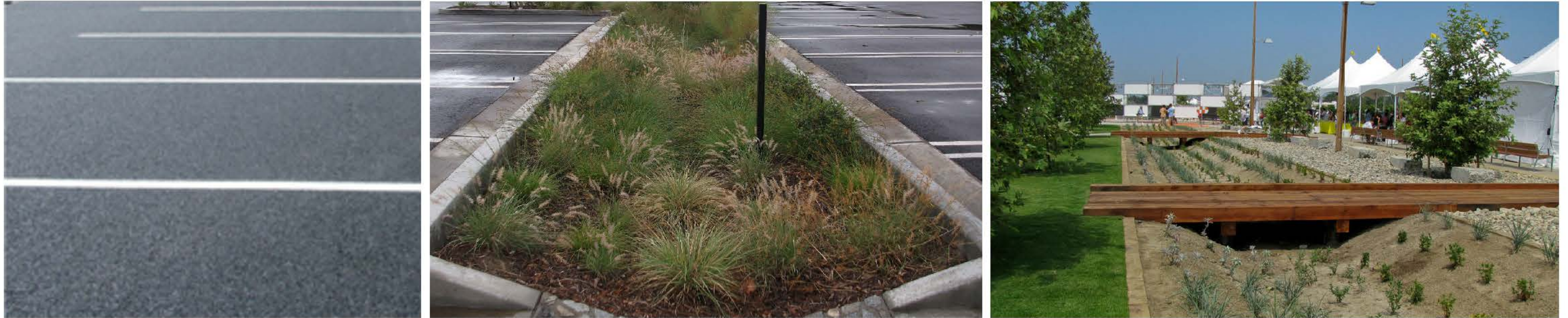
Parking lot & bioswale
