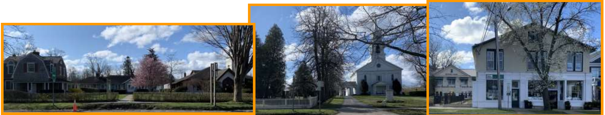
South side of Main Street, left to right, No. 2463 Main St., 32 Hull Ln., 2429 & 2415 Main St.
