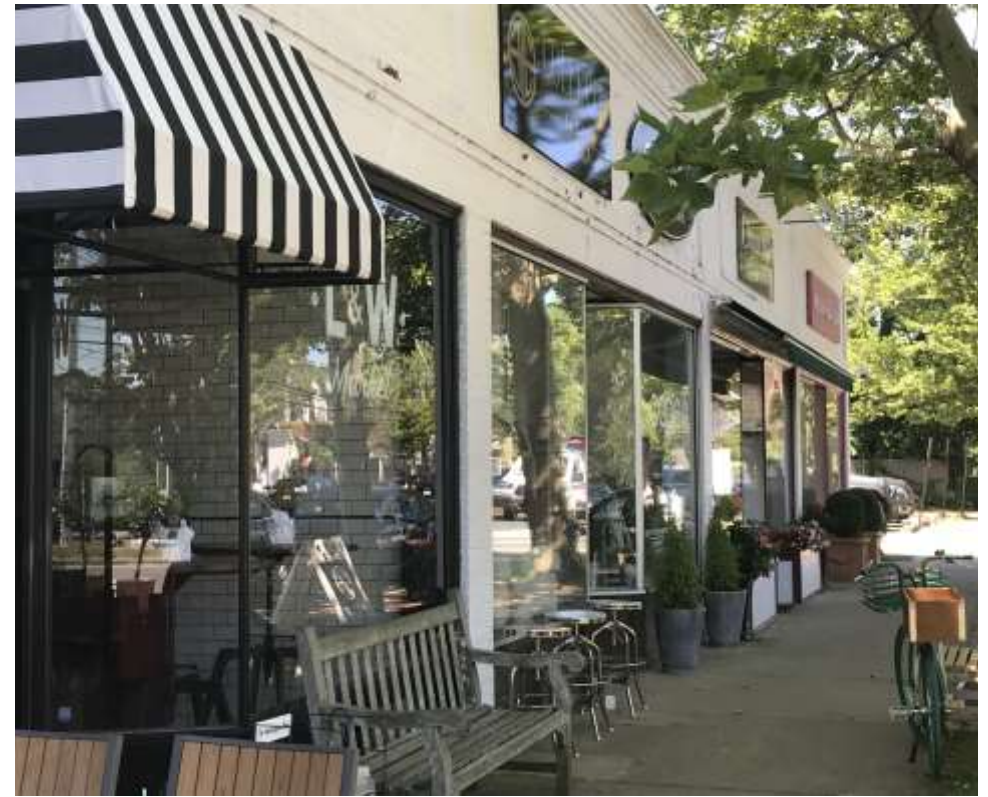
These four one-story brick buildings, built by Kenneth Chester in 1928, are now home to L&W Market, Capelli Hair Salon, Churchill Wines & Spirits, and Helen Ficalora Jewelry. The contractor, Topping and Griffing, and stonemasons, Ruppel and Chester, were local.
