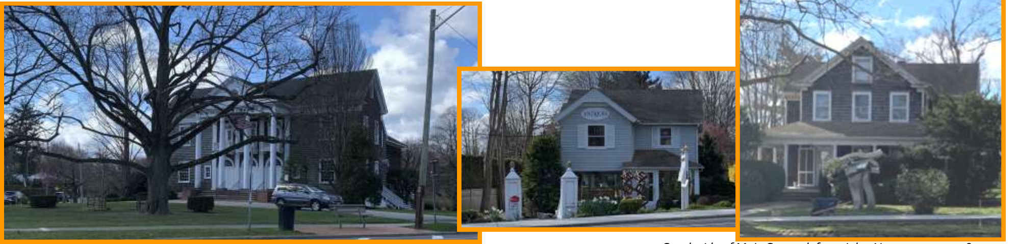
South side of Main Street, left to right, Nos. 2357, 2309, & 2297.
