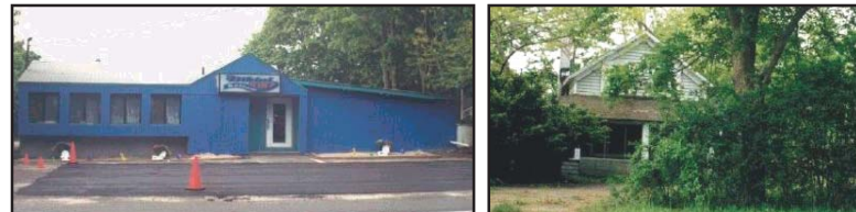
The Bikini Bottom nightclub and adjoining dilapidated property on Montauk Highway in Westhampton present nuisance problems in a residential neighborhood. This property assemblage represents a redevelopment opportunity to facilitate community housing opportunities in proximity to schools, services, and public transit.
