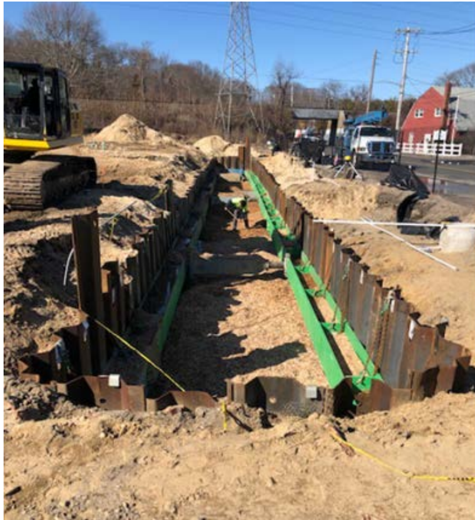
Figure 1-6 Nitrex PRB just prior to completion
