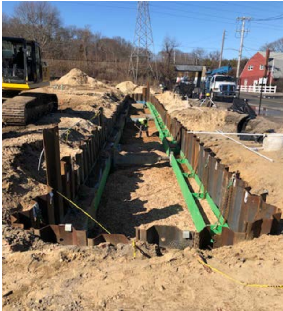
Figure 1-6 Nitrex PRB just prior to completion
