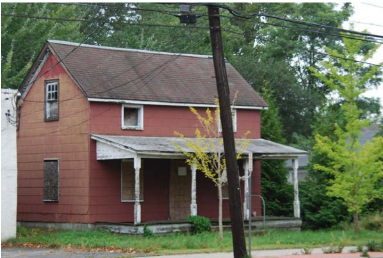
Photos of 43 Flanders Road Source: NP&V Photos (September 30, 2015)
