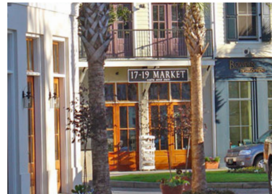
Precedent images of buildings allowing co-working and creative class space without compromising quality of a street experience and walkability.
