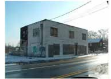
Site Photograph 2 Former Building
