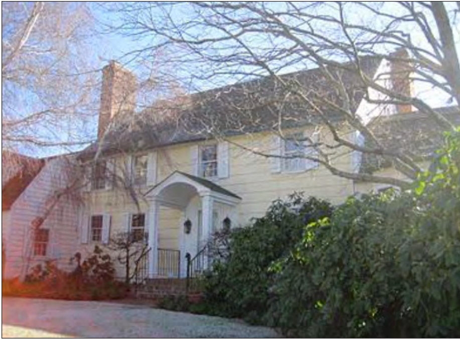
WM-53 186 Crescent Avenue
