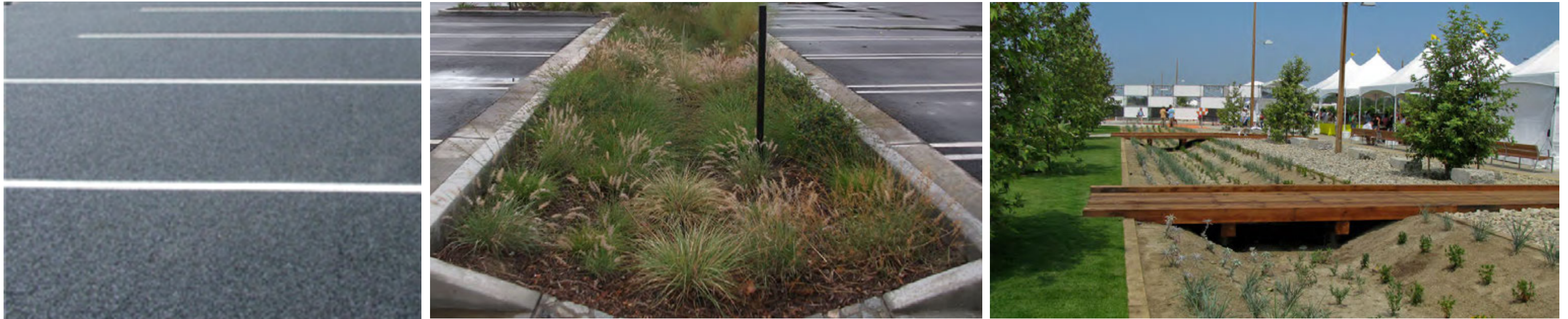
Parking lot & bioswale
