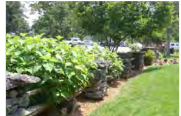
Fence with masonry posts and wood rails screen
