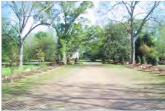
Permeable pavers with natural landscape edges
