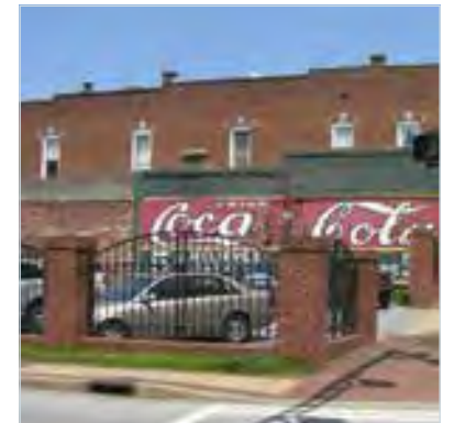
Brick wall with metal fencing
