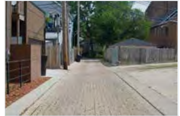
Permeable pavers in alley
