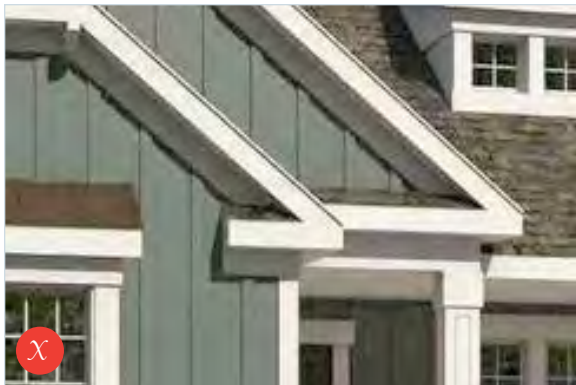
Oversized fascia without terminating eave moulding; eave return roof is not hipped
