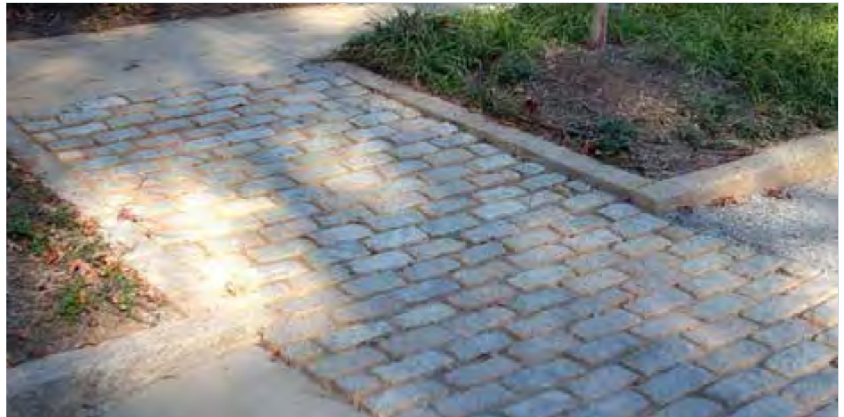
Stone paving with permeable gravel joints
