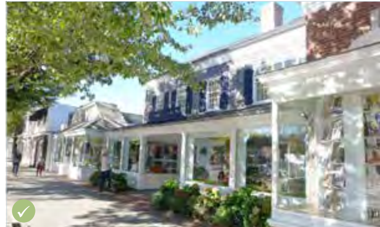
East Hampton This building presents a single-story filled-in porch in front with the primary two-story massing behind . The different buildings' primary masses sit in various planes within the frontage zone which leads to a casual streetscape .
