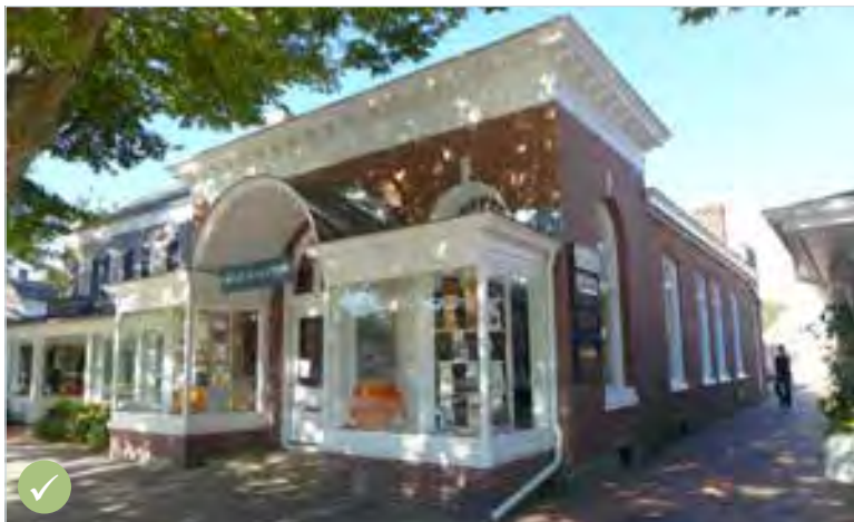
East Hampton This pair of buildings undulate relative to one another, creating a more organic pattern.
