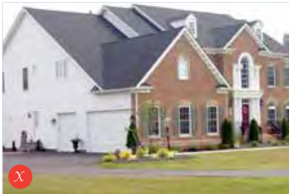
Material transition at outside corner
