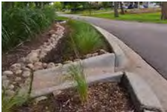
Curb cut draining to bioswale
