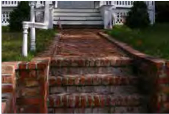
Stairs and wall addressing grade change
