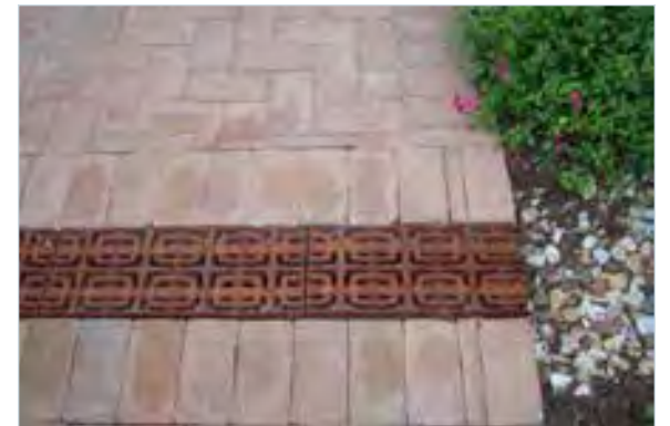
Trench drain and pavers
