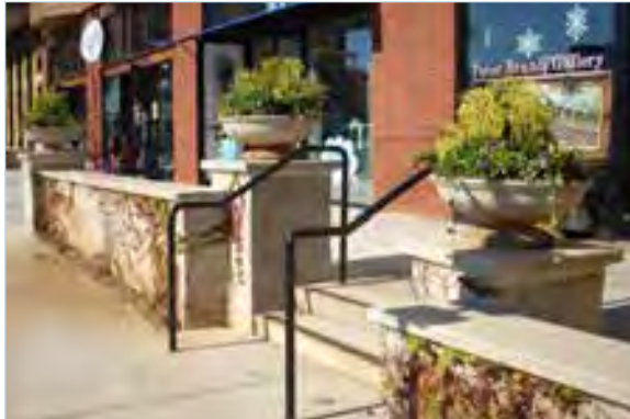
Stair and wall addressing grade change
