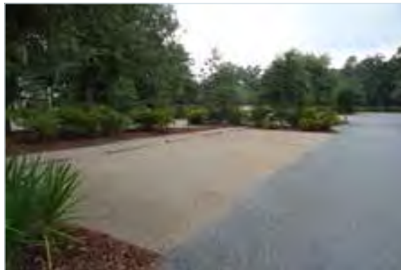
Permeable parking pads
