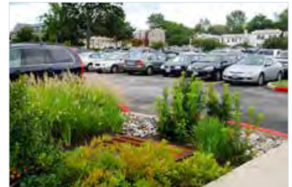
Rain gardens within lots to collect stormwater
