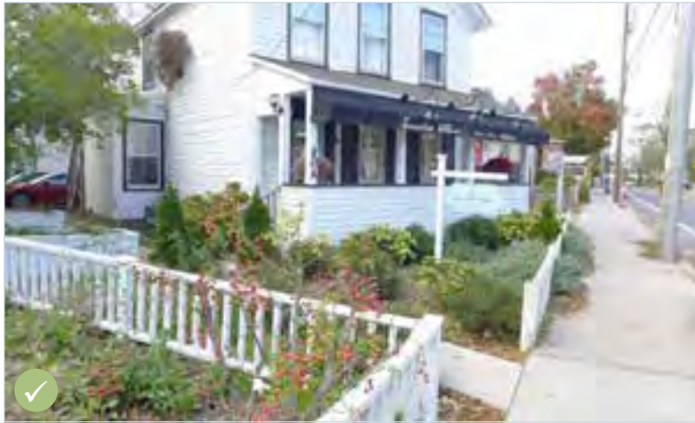
Sag Harbor A moderate setback can allow for nice planting while still having the building address the street .
