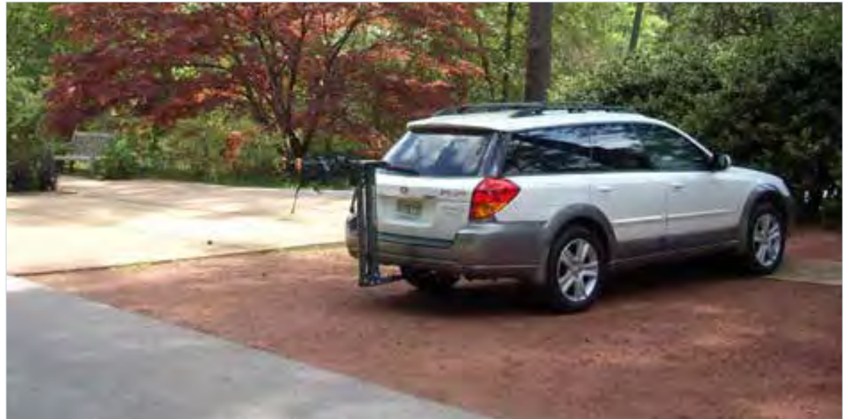
Permeable surface for car parking
