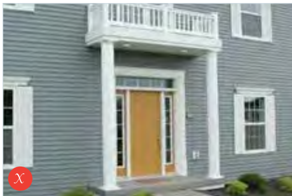
No pilaster at supporting porch wall & columns are too thin and/or too tall
