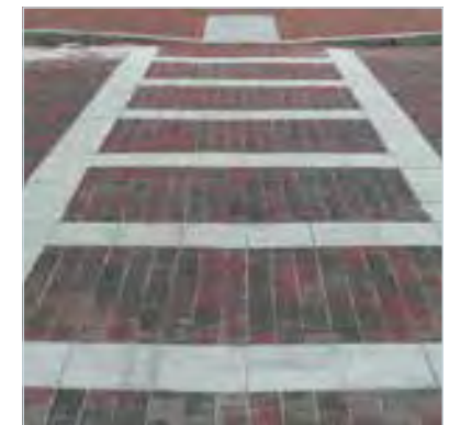
Brick and granite crossing
