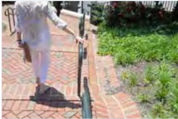
Runnel placed adjacent to exterior stairs
