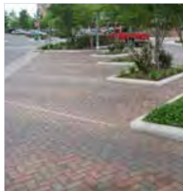
Brick pavers in parking lot
