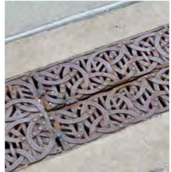
Close up of decorative Trench Drain
