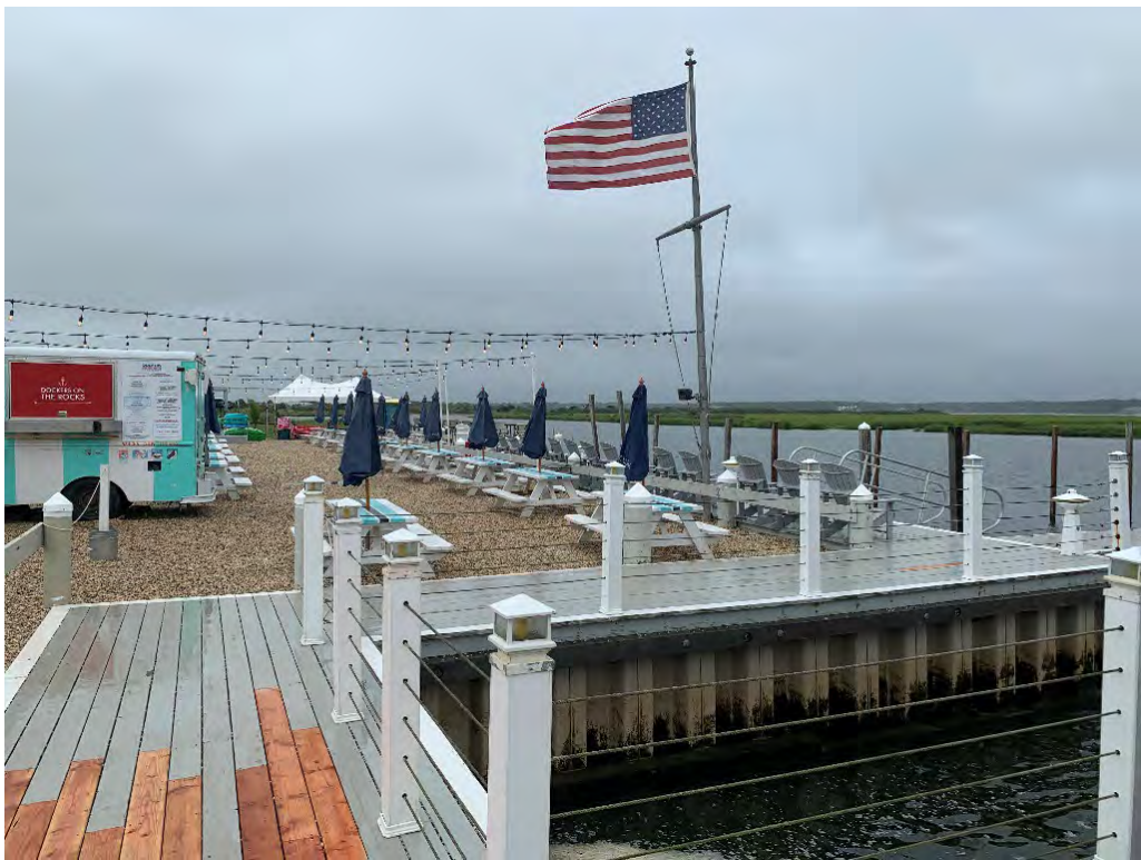
Photograph No. 12 – View of eating area and walkway along bulkhead with access to floating dock, facing west. (Photograph taken August 5, 2021)
