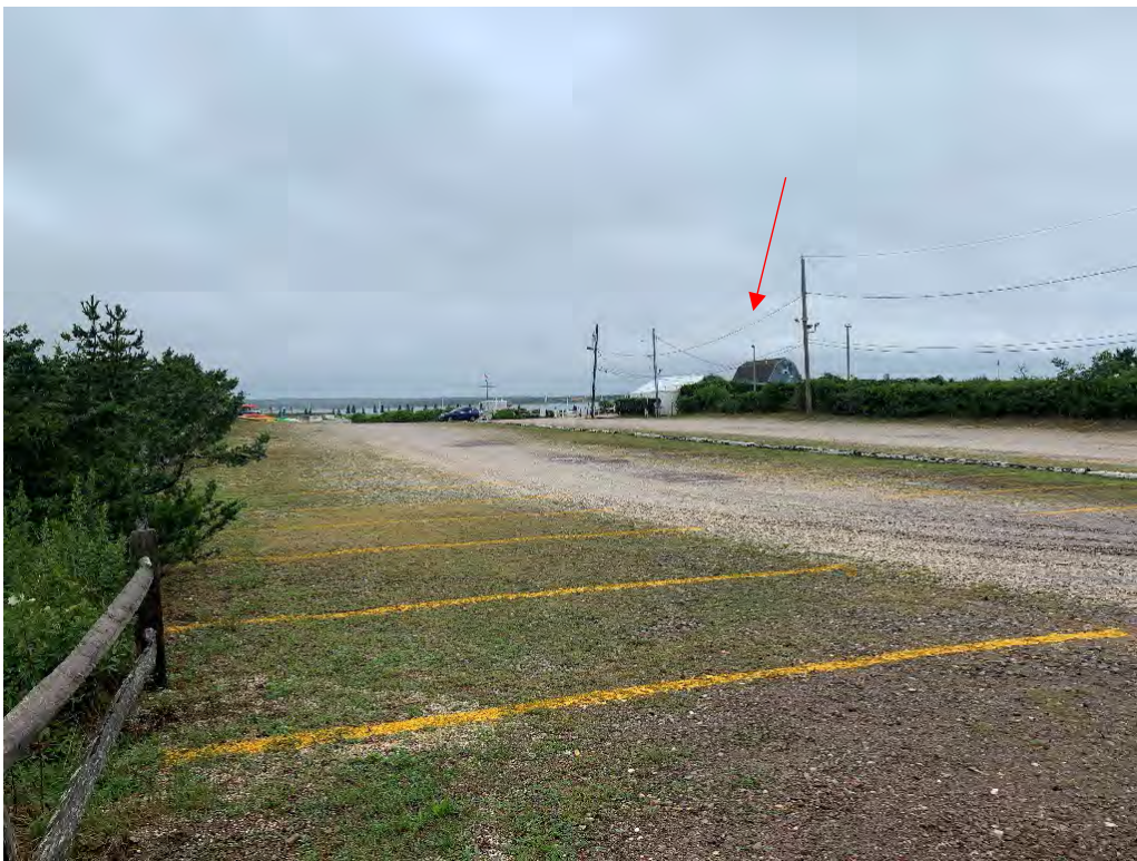
Photograph No. 4 – View of surface parking lot southwest of existing restaurant/bar, facing northeast. Existing restaurant/bar structures (shown at red arrow) and existing overhead utility wires present with vegetative screening in eastern portion of photograph. Existing Town-owned open space visible in western portion of photograph. (Photograph taken August 5, 2021)
