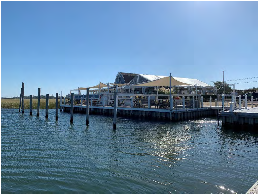
Photograph No. 11 – View from floating marina dock of existing bulkhead with restaurant/bar and associated awning, tent, and deck beyond, facing southeast. (Photograph taken October 1, 2020)
