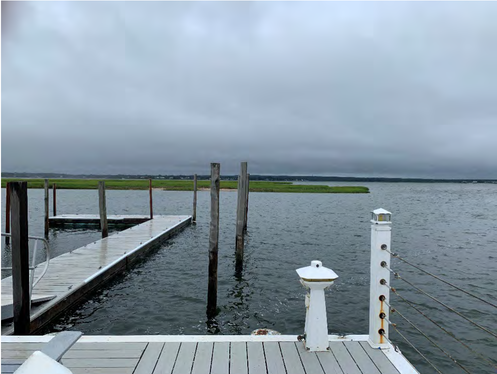
Photograph No. 16 – Representative view north of subject property, facing north across Shinnecock Bay. (Photograph taken August 5, 2021)
