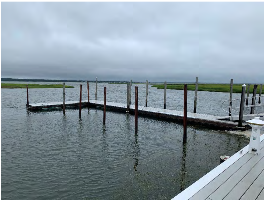
Photograph No. 14 – View of floating dock, facing northeast. (Photograph taken August 5, 2021)
